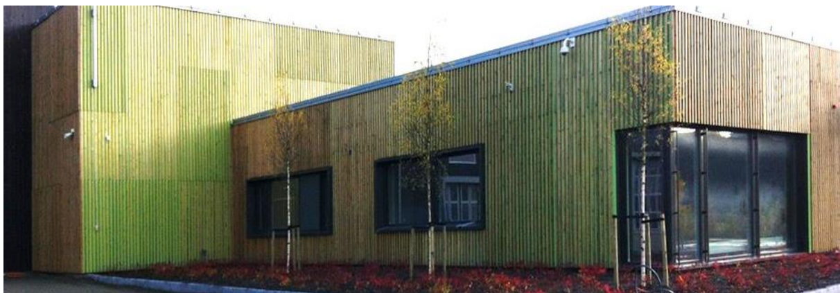
Figure 8: Wall installation at Sandmoen fire station, Trondheim, by Edith Lundebrekke. Collected from edith.no/project/fire-station-trondheim .
