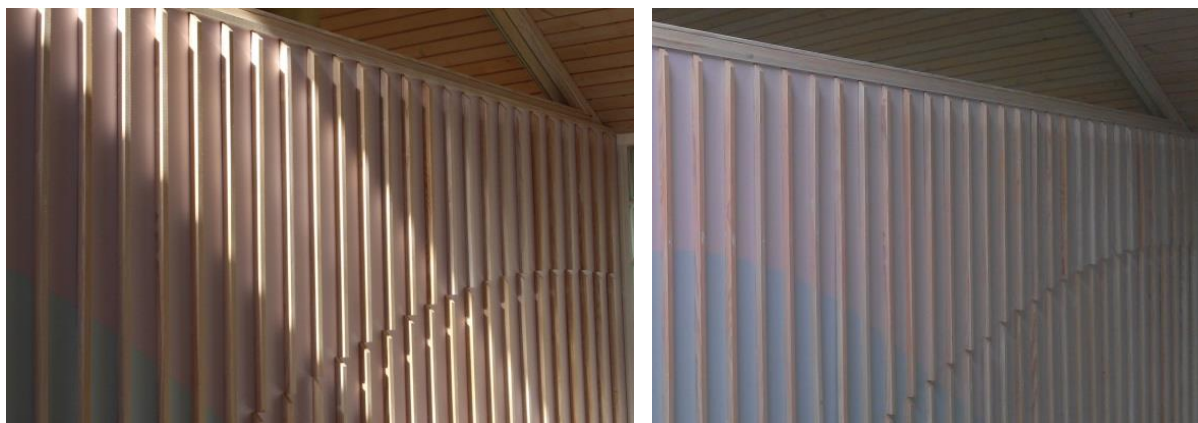
Figure 10: A relief wall in the detached house, Steinåsen 44b in Trondheim, designed by the author. Pictures taken with sunlight and clear sky to the left, and overcast sky to the right. Photos B. Matusiak, 2015.
